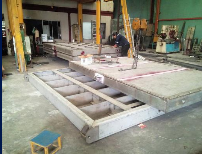
Water gate fabrication
